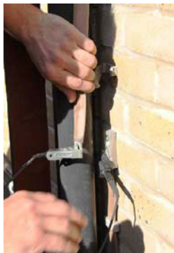
Two pole test
