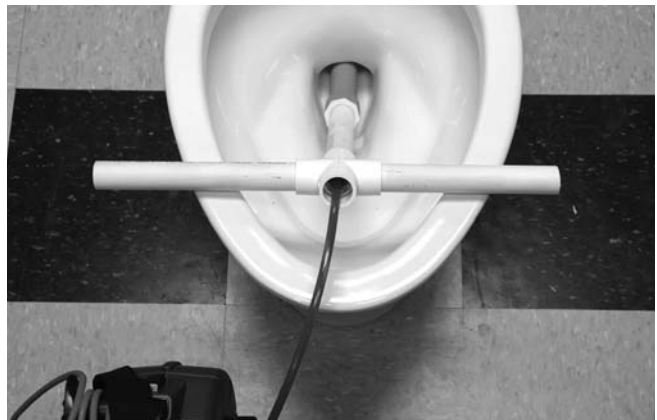
Figure 24 – Using A PVC Guide Tube
