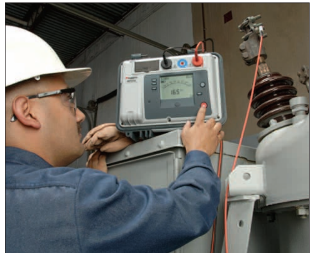
Delta wye transformer being testing with a MIT520/2
