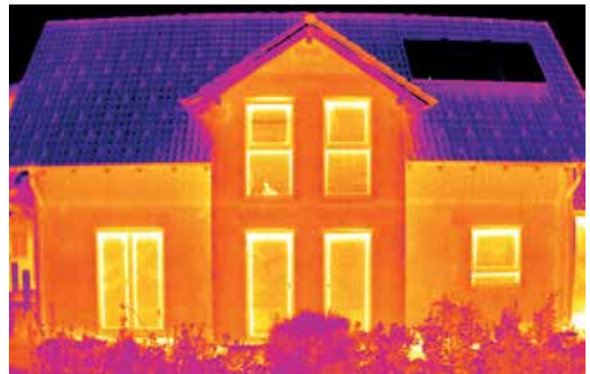
Complete building front in a panorama image.
