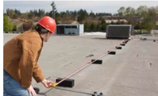
Measuring long conduit runs.
