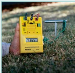
Check resistance between earth and grounding rod.
