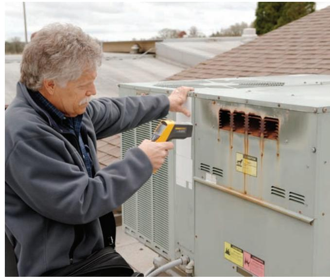
Testing roof-top refrigeration system with a Fluke 561 Infrared Thermometer.
